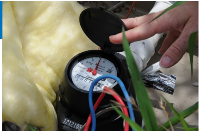
Figure 6. Monitoring irrigation water use with a water meter can provide an alert in the event there is a leak in the system or a solenoid is open.
